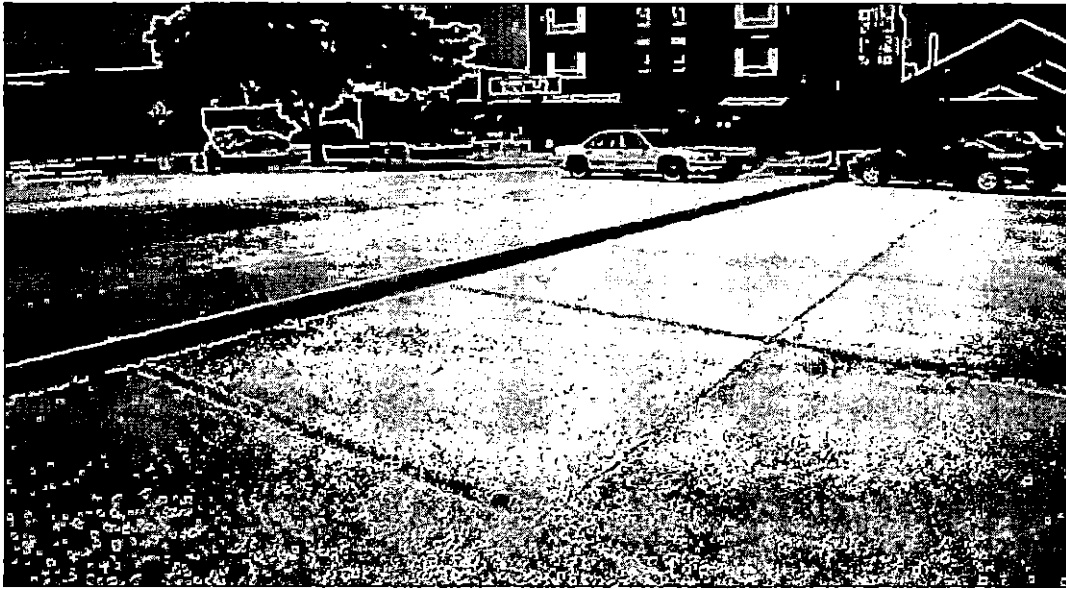
Figure 15. Pervious Concrete Installed in Lincoln, Nebraska.
