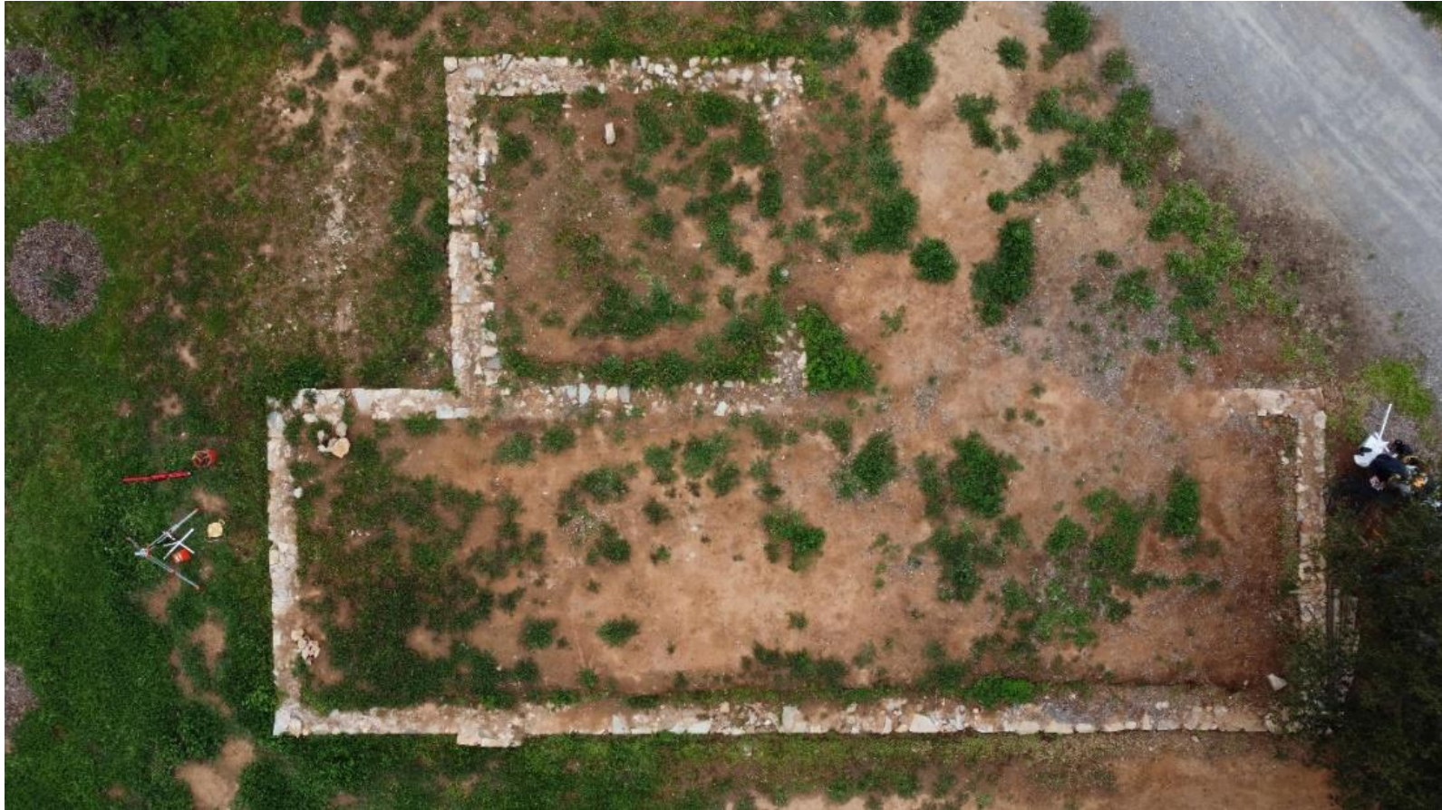
Figure 3. Drone photo of the building foundation. Photo courtesy of Palomar College.
