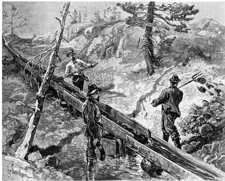
Figure 7. "The Sluice", Illustration showing miners feeding material into a long tom sluice (uppermost worker with shovel) and removing larger rocks with a "sluice fork" (right-side worker). This illustration was published in The Century illustrated monthly magazine in Jan 1883 (Sandham, 2010; public domain).
