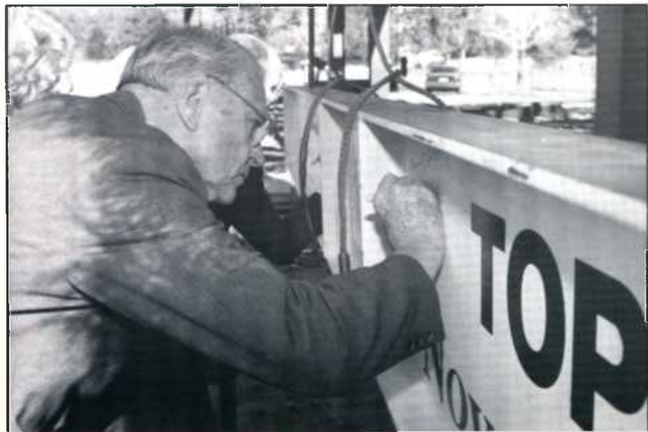
ON THE BEAM —Major contributor Robert V. Fullerton signs his name to the beam that was hoisted up during the topping out ceremony for the Visual Arts Center on Nov. 28. The art museum part of the complex was named after Fullerton, and is now less than $20,000 short of its $760,000 goal in funding. An American flag and a Christmas tree sat atop the beam, a tradition in construction projects that began around the turn of the century. The museum is a 4,000-square-foot building with two galleries connected by a colonnade, the visual arts center a 58,510-square-foot classroom, office and research facility.
