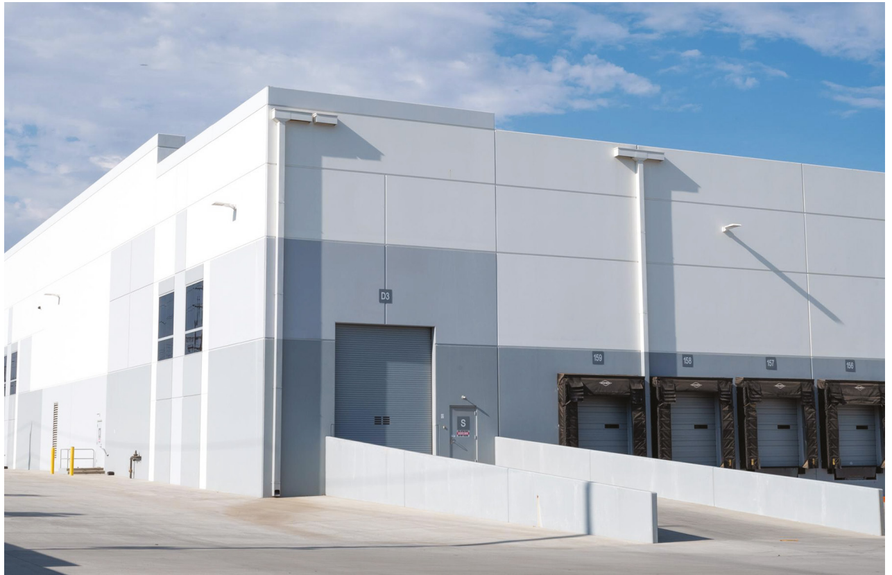
Garages remain closed until trucks arrive at a Bloomington warehouse on August 26, 2022. This facility sits directly across the street from Zimmerman Elementary School which will be demolished and relocated due to the construction of the Bloomington Business Park Specific Plan approved by San Bernardino County in late 2022. Environmental groups are suing the county for violating the California Environmental Quality Act. (Aryana Noroozi for Black Voice News Newsroom / CatchLight Local, August 24, 2022).
