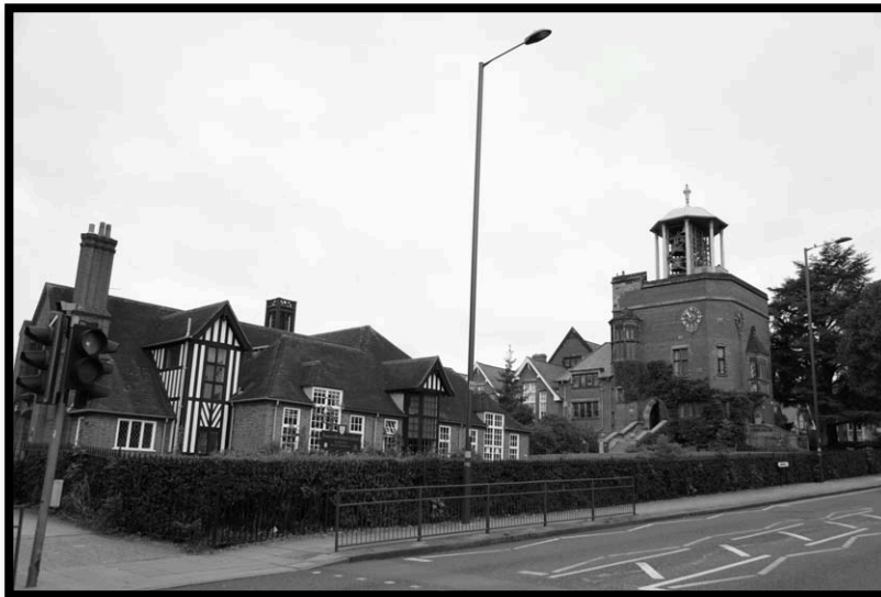
Figure 2-3: Row houses and pre-school & primary school in Bournville, England. England. Photos by author.
