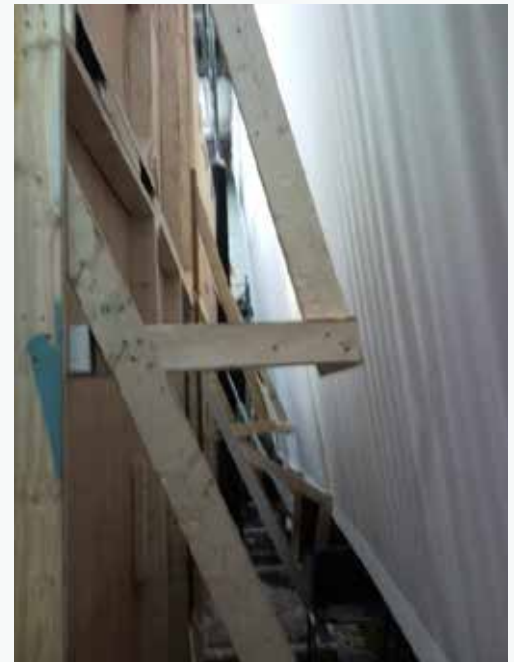
Figure 11. 2 x 4 Trusses in School Play Set.
